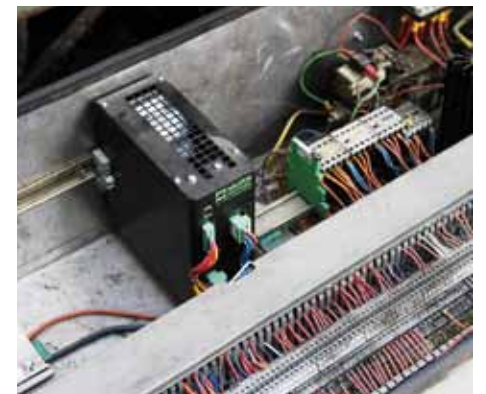
MB Cap for Buffering Voltage Drops
